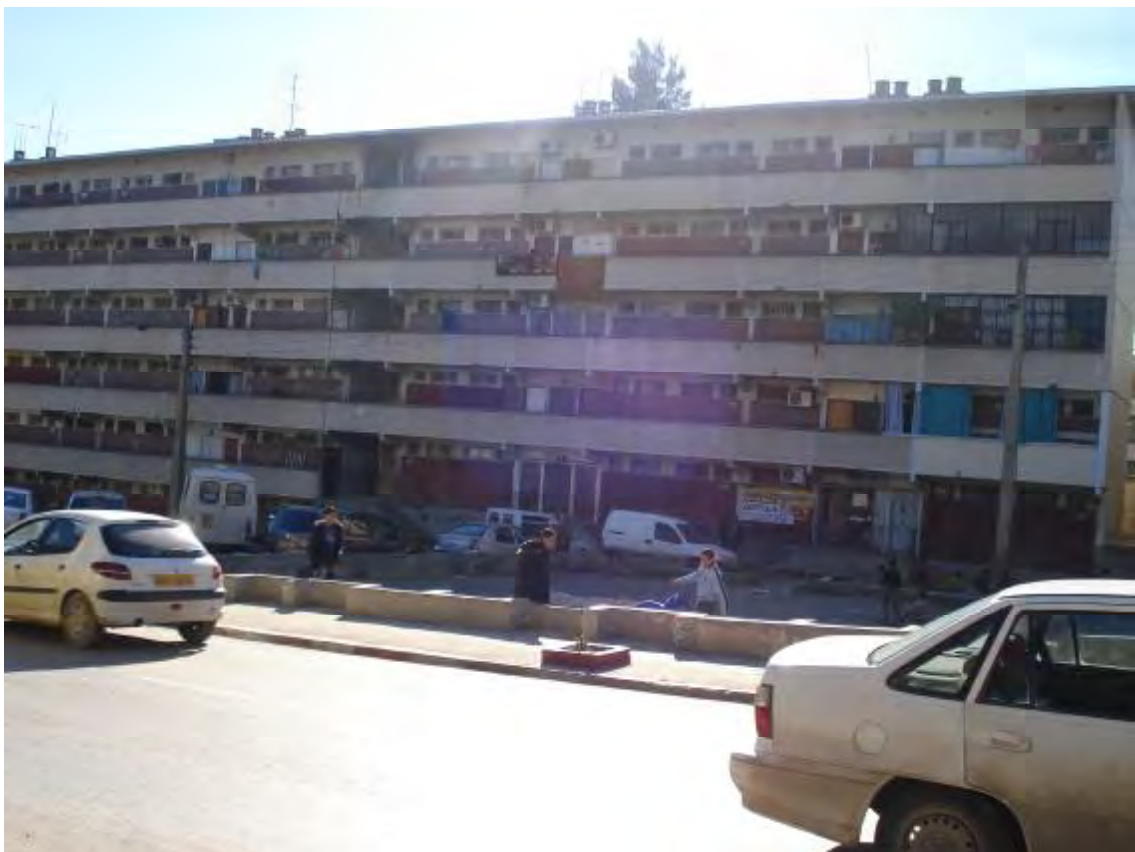
Figure 15: View of the “street in the air development”, Cité les Chasseurs, Constantine (the author).
