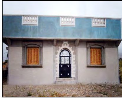
Photo III.20 & Photo III.21 & Photo III.22 : Logement Rural à Tlemcen.
