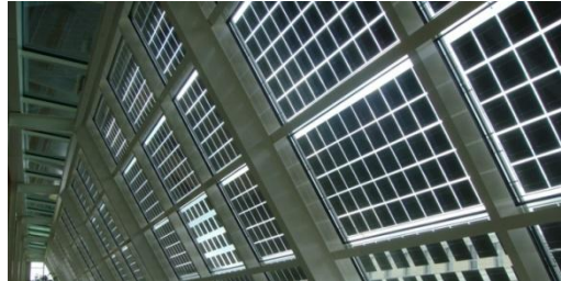
Figure II.7. Vitrage photovoltaïque
