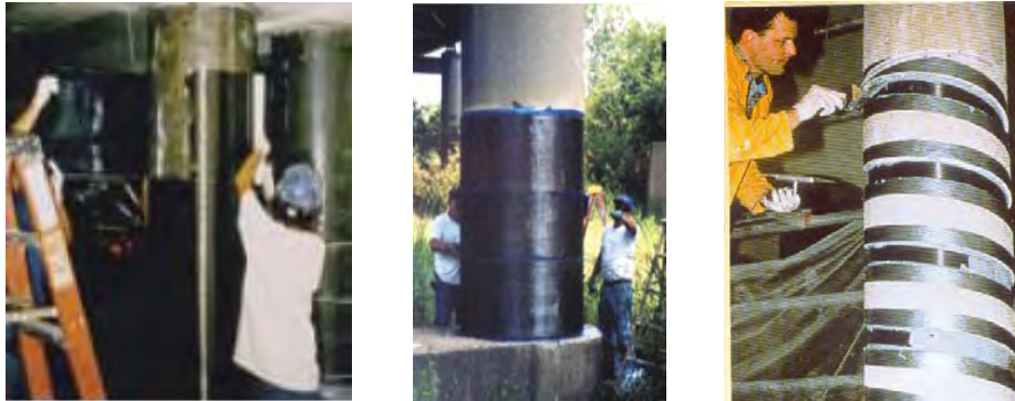
Figure I-14 : Stratification au contact.
