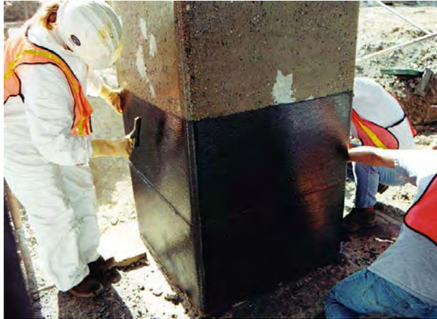
Figure I.2. 6: Confinement de colonnes (Pantelides et al. 2002)
