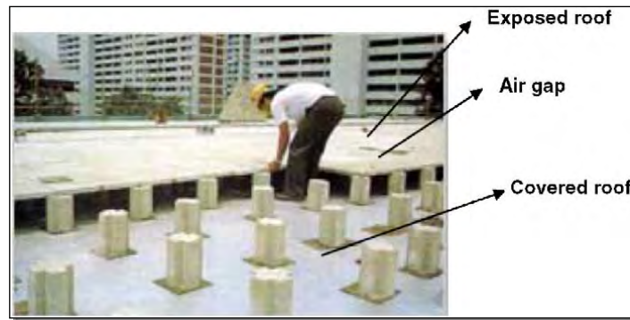
Fig. IV. 8 : Secondary roof system construction. (Source: Wong N.H. & Li S. 2007).
