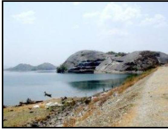
Figure 5.10 Barrage Béni-Haroun. (coyne-et-bellier, 2008)
