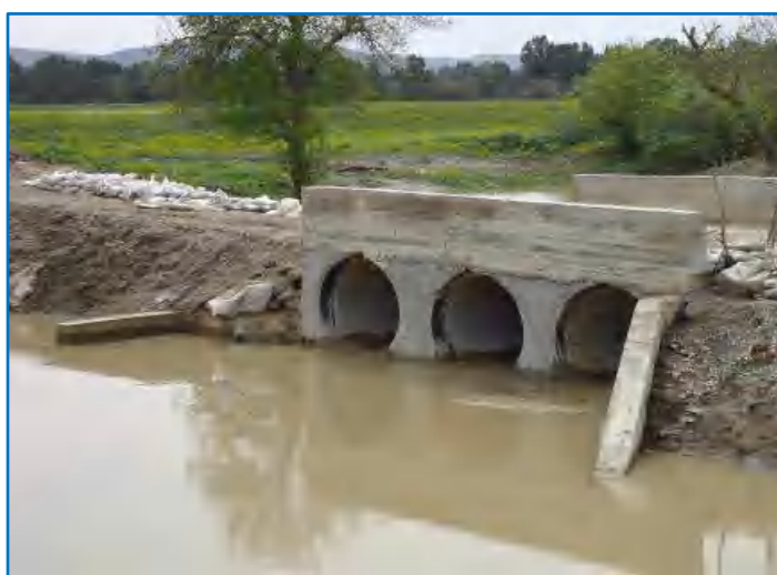
Photo 26. Passage busé (3×1000) digue 6 route Ain Khiar (ONID, 2012)
