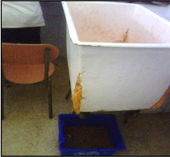
Figure 11 Bacs fissurés
